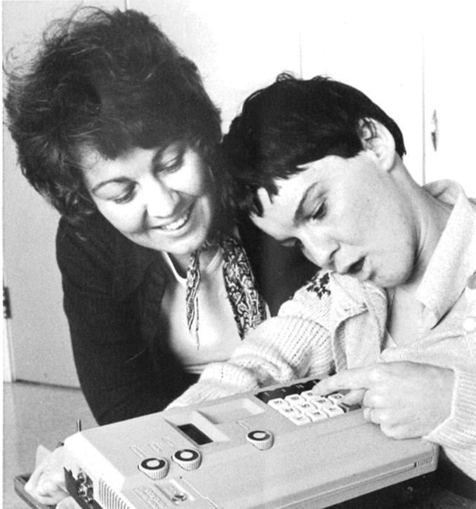
Nancy and Margaret with a HandiVoice 120. The HandiVoice 110 & 120 were the first portable, commercially available AAC systems with synthesized speech output.
